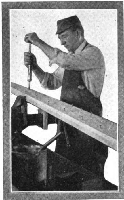
Fig. 3—Screwing the laminations of the sill together
